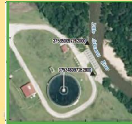
Groundwater Recharge Source: USGS: 2016-5042
