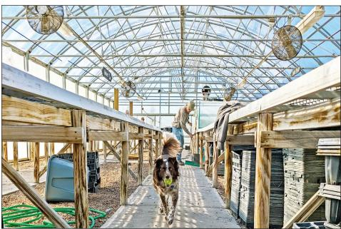
Clockwise from top left: In January the crew from Preferred Builders removed the deteriorating double layer of polyurethane. New bracing and a ridge cap were added to support the Lexan thermoclear plastic sheets. Rosie, the greenhouse dog, plays fetch while volunteer Gerry Selzer prepares the space for spring.
